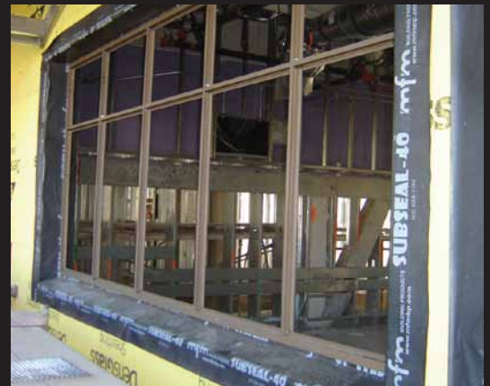
SubSeal bonds aggressively to poured concrete and other building materials. It is fully adhered to the substrate to eliminate movement of water under the membrane.
