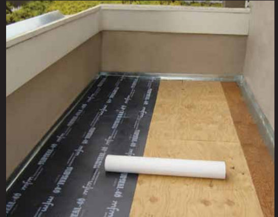
SubSeal is an excellent choice for waterproofing balcony decks and other surfaces that will be finished with concrete.
