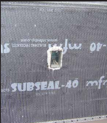
Apply polyurethane sealant when terminating all exterior penetrations.
